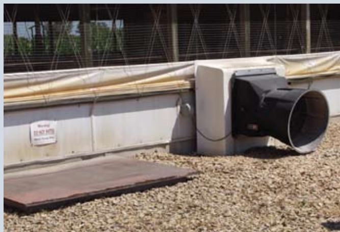
Pit ventilation in a finishing facility
